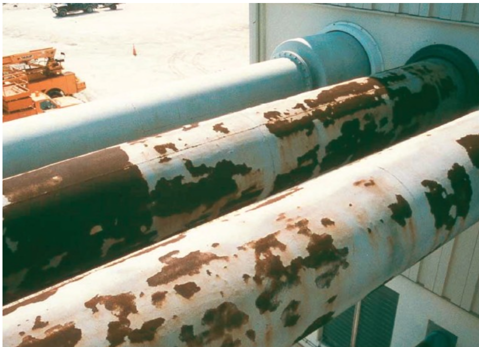
Figure 52 Corrosion on High Temperature Pipelines at an Air Force Facility 42
